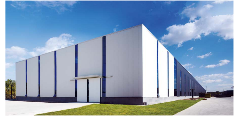
柏博森丽彩晶®聚氨酯冷库板生产车间 | Production Workshop of Berbson Colorspar® PU Cold Storage Panel
